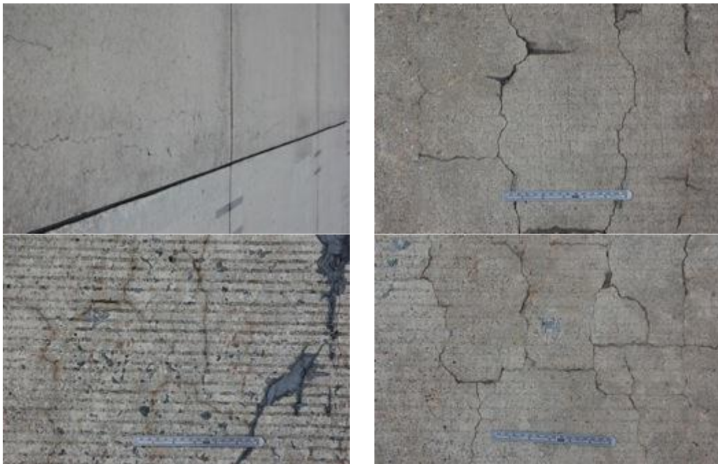
Figure 13: Airport VI Visual Survey of Taxiway Bravo
