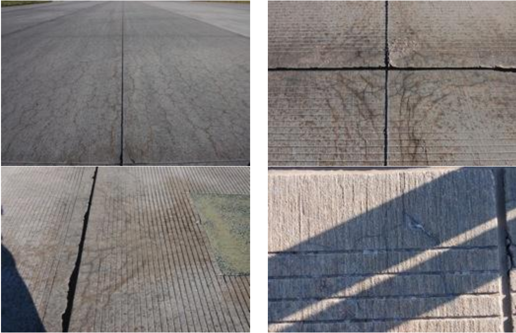
Figure 7: Airport IV Visual Survey of Taxiway Echo 5
