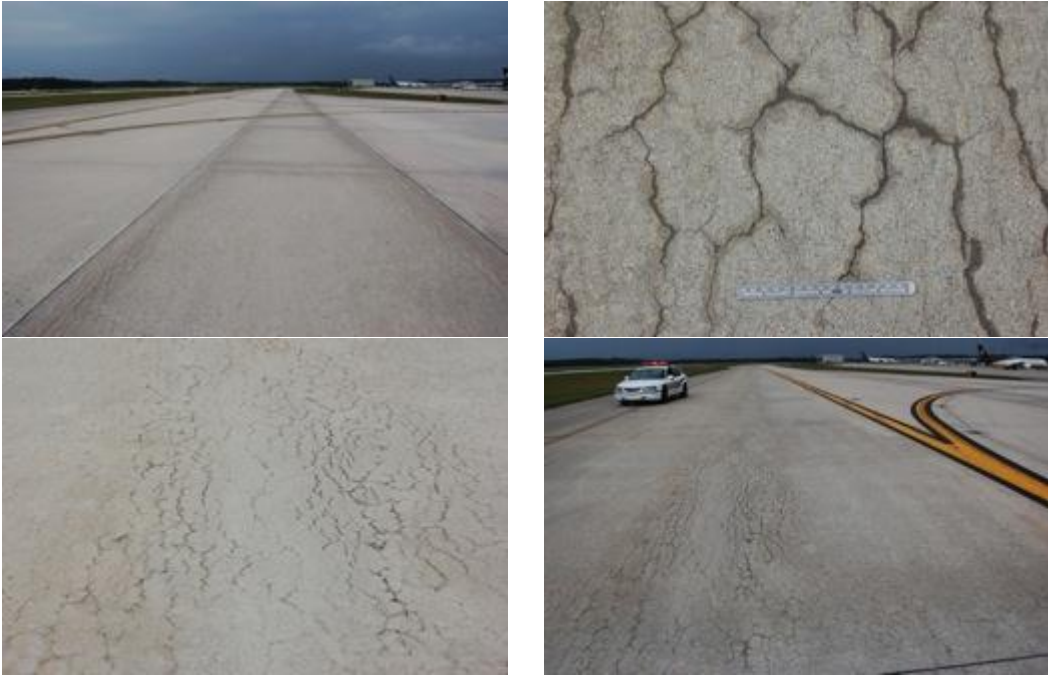
Figure 14: Airport VI Visual Survey of Taxiway Foxtrot
