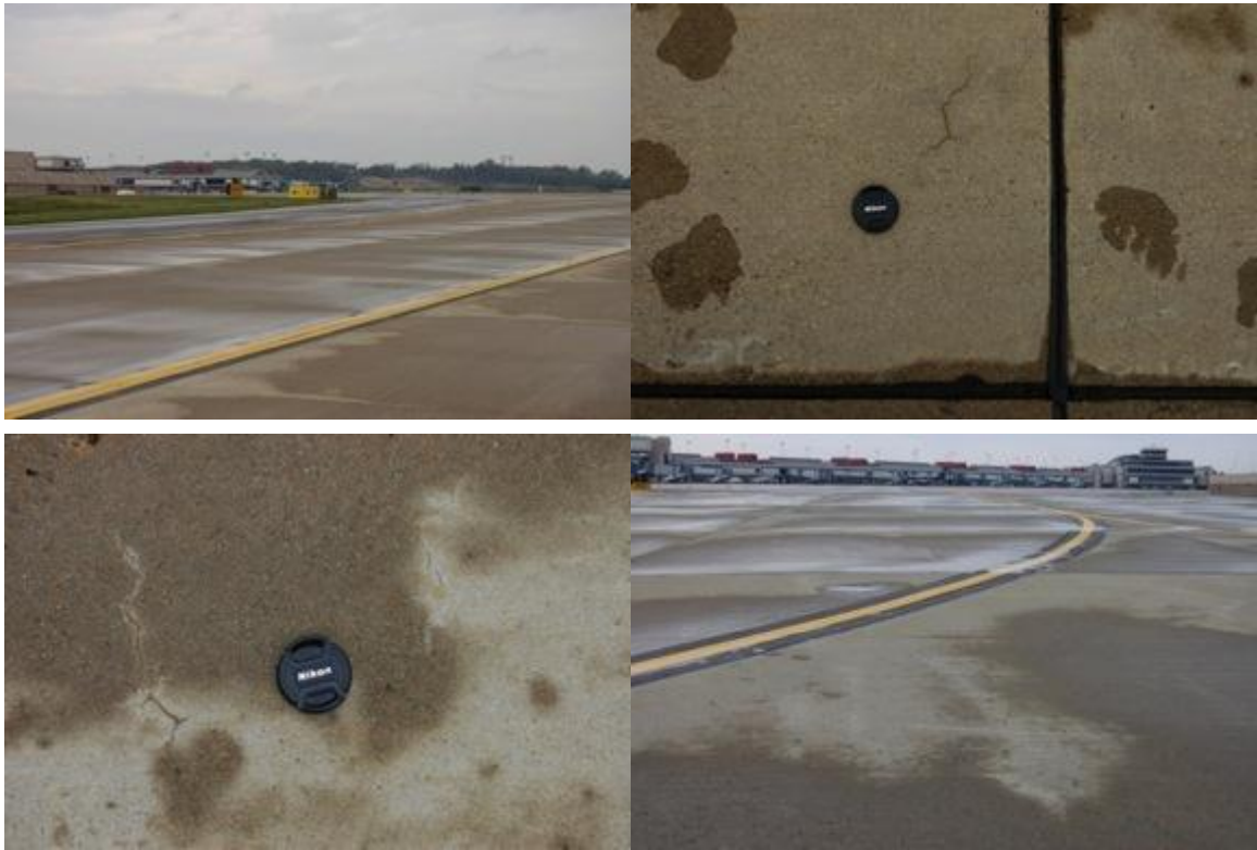
Figure 2: Airport I Visual Survey of Taxiway Tango
