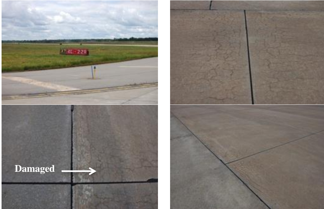
Figure 12: Airport V Visual Survey of Damaged Sections
