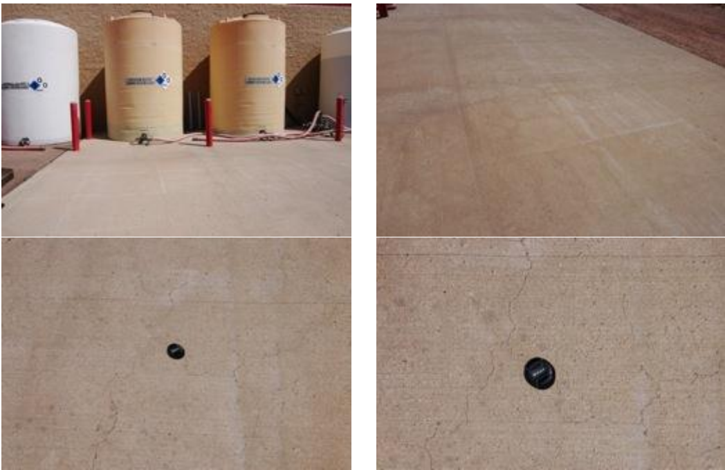
Figure 10: Airport IV Visual Survey of Deicing Pad
