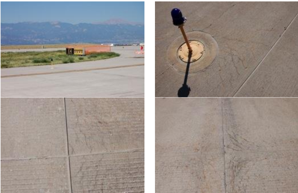
Figure 8: Airport IV Visual Survey of Taxiway Echo 4
