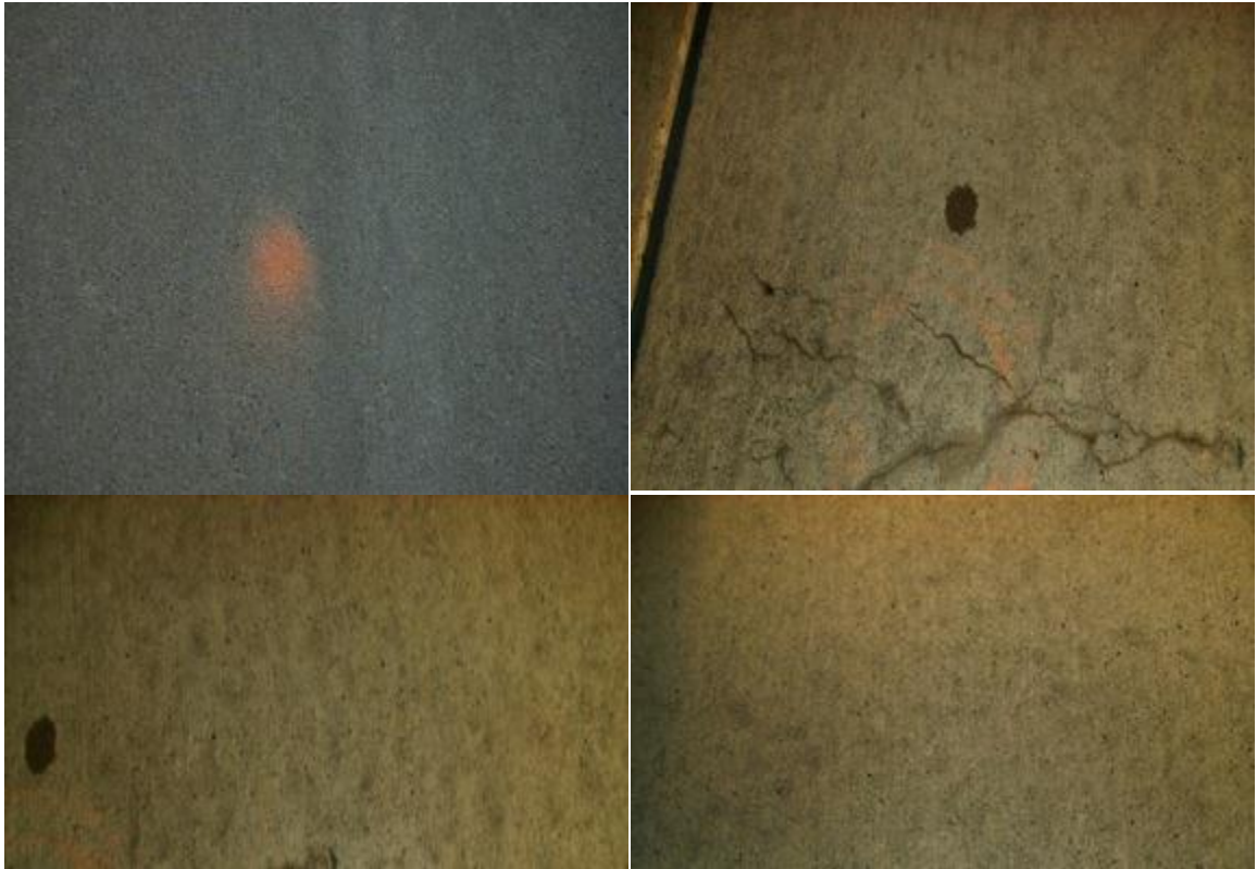
Figure 3: Airport I Visual Survey of Taxiway Victor
