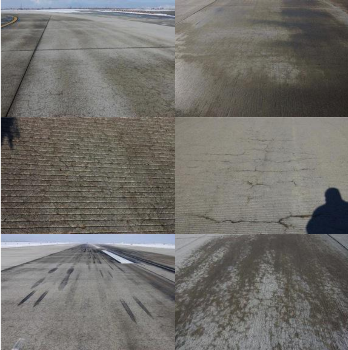
Figure 5: Airport III Visual Survey of Runway 16R/34L
