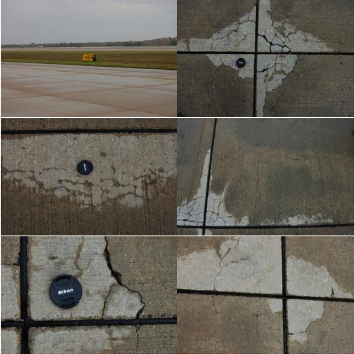
Figure 1: Airport I Visual Survey of Taxiway Echo
