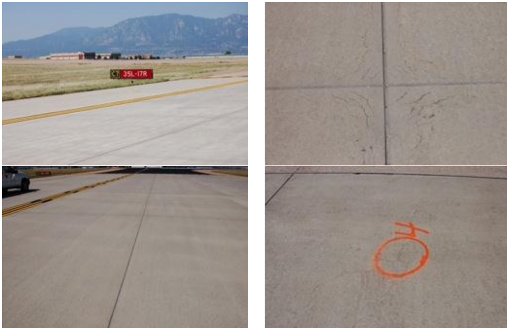
Figure 6: Airport IV Visual Survey of Taxiway Charlie 7
