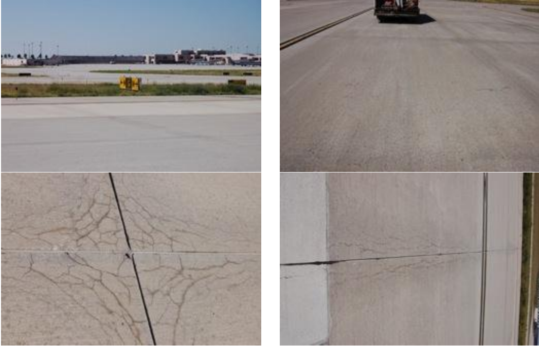
Figure 9: Airport IV Visual Survey of Taxiway Golf
