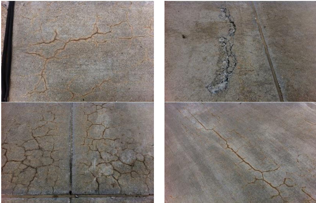
Figure 16: Airport VII Visual Survey Representative Pictures
