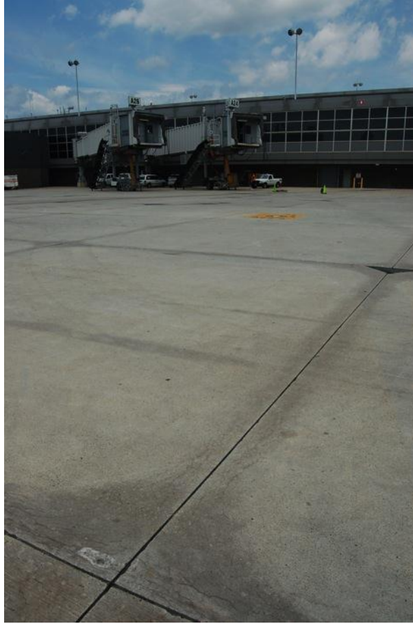
Figure 18: Airport VIII Visual Survey of the Apron
